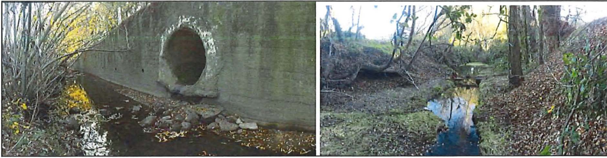
Figure 12. Concrete retaining wall with 48" stormdrain outlet on opposite bank from the Penngrove Community Park (left) and typical channel near the downstream end of the baseball field in the park (right).
